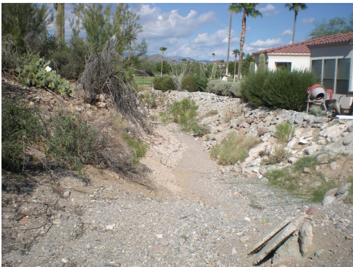
Queen Valley flood control improvement area
