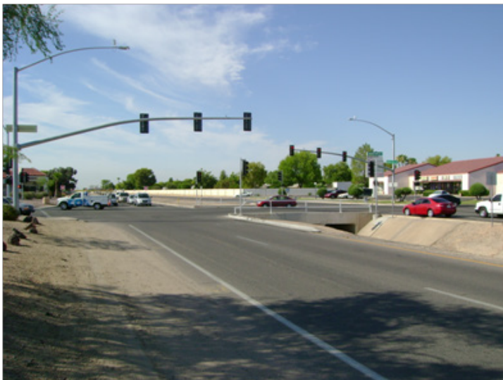
Union Hills/99th Avenue traffic signal upgrade
