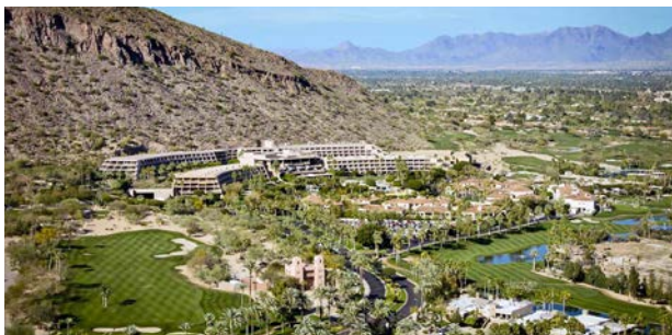
ADA Facilities Assessment, Site Field Surveys and Upgrades @ The Phoenician Phoenix, Arizona
