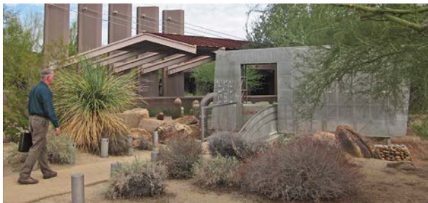
Scottsdale Water Campus Buildings Remodel Scottsdale, Arizona
