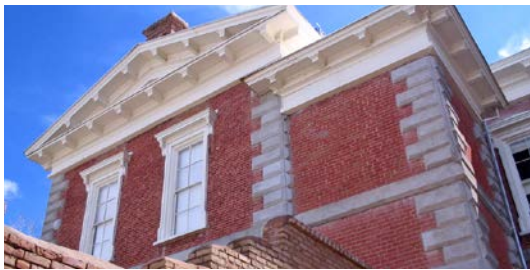
Tombstone Courthouse State Historic Park Historic Building Renovation
