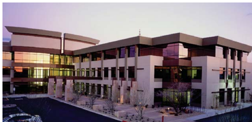
Pegasus Office Building and Data Center Complex
