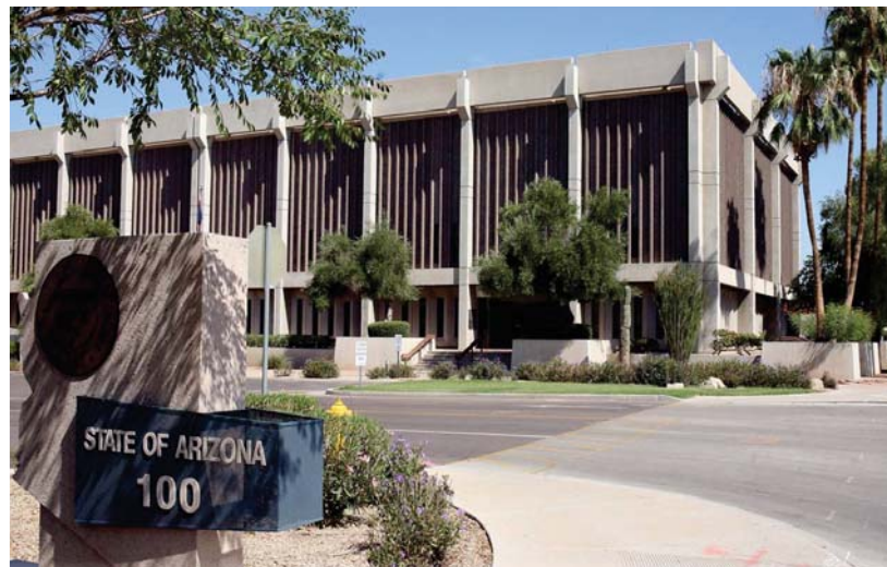
Arizona Department of Administration Data Center
