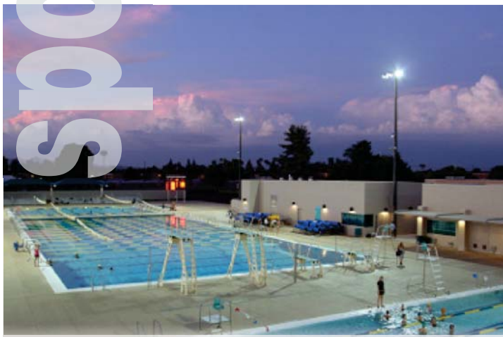
City of Mesa Kino Pool Renovation
