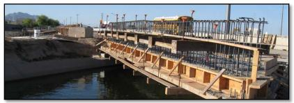
The improvements consisted of structural additions to bridges, overlaying the bridge decks with asphaltic concrete, and widening of the existing roadways north and south of the bridges. Other project improvements were curb and gutter, sidewalks, street lighting, drainage improvements within the right-of-way, landscaping, utility extensions, and signing and striping.
