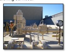
pumps, valves, surge tanks, a flow meter, chlorine analyzer, motor control centers, generator (back-up power), air compressor, telemetry, security gate, sound/perimeter wall, pump starters, relays, automatic transfer switch, switchgear.
