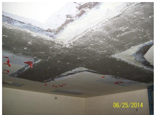
After application of Carbon Fiber Material
