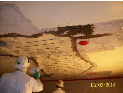
Epoxy applied over exposed rebar
