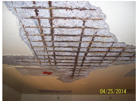
Removal of deteriorated concrete
